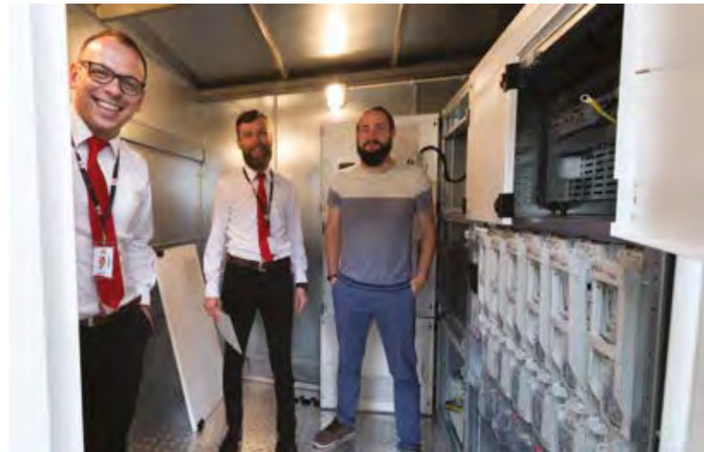
FAT tests before a switchgear delivery to a final customer
