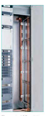
The vertical PE and N busbars are located on the right side of the cable compartment.
