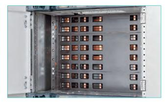
Distribution busbar system, protected against accidental contact (IP20B)
